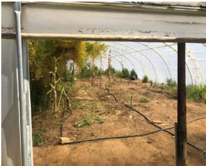
The growing tunnel (offered by a faculty member) before the project began
